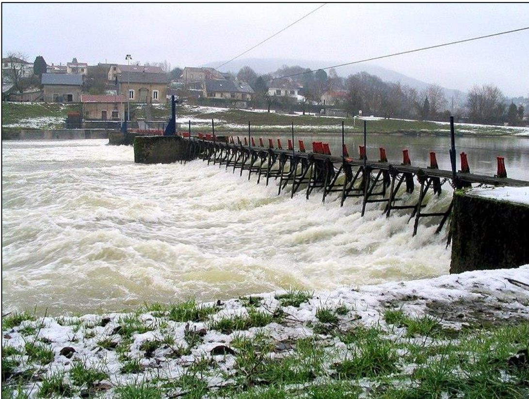
Figura 1-14 Diga Weir, Francë (Roose, 2004)
