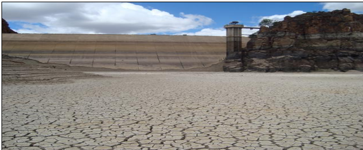
Figura 1-16 Diga Beaufort West (Head, 2017)
