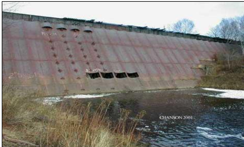
Figura 1-11 Diga çeliku Red Ridge, ndërtuar 1905, Michigan (Miller, 2001)
